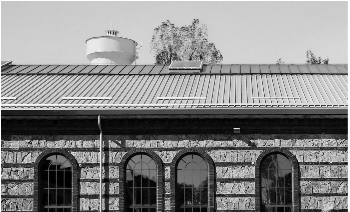
Picture n° 5: roofing made with Isolpack Lithos 5 fire certified sandwich panels.
